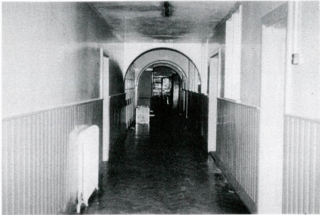
The Corridor leading to the Assembly Room and classrooms
